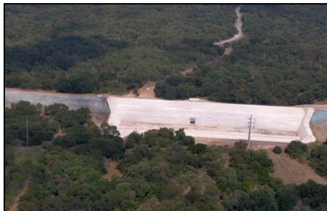
Salado Dam 15R is an example of BRWM structural improvements for flood control.
